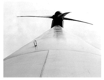
Figure 6: One of the loop antennae for the lightning sensor system placed on the tower of a 1 MW wind turbine at the power plant Avedøreværket in Copenhagen.
